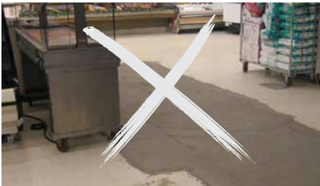
A Vacuum Plumbing System eliminates a saw cut floor
