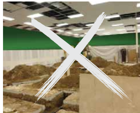
A Vacuum Plumbing System eliminates the mess associated with trenching or cutting of the slab
